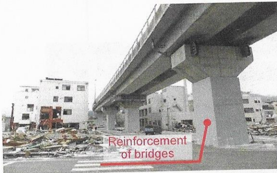
Condition of a bridge after the Great East Japan Earthquake (seismic reinforcement was completed)
